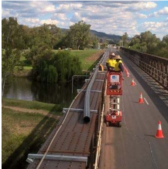
Figure 1: Installation of temporary poly main
